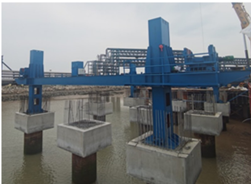
图 2 支腿驻位桩帽 Fig. 2 Supporting legs standing on pile caps
