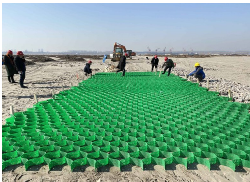
图2 铺设中的蜂格柔性三维网格 Fig.2 Flexible 3D grids with honeycomb structure during installation
