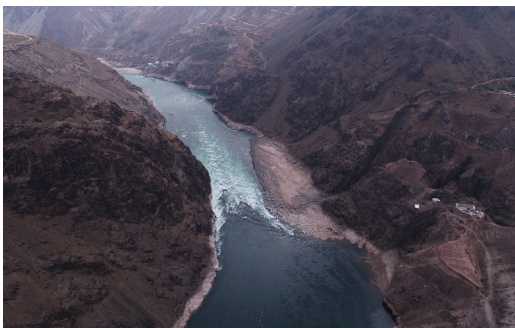
图8 金沙江白鹤滩电站库尾滩险流态 Fig. 8 Dangerous flow pattern of tail beach of Baihetan power station on Jinsha River
