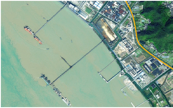
图 3 岑港港区老塘山岸线复式布局优化 Fig. 3 Compound layout optimization of Laotangshan shoreline in Cengang port area
