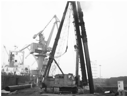
图4 陆上打桩机沉桩
