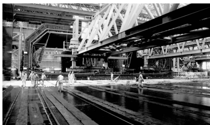
d) 浇筑台座钢筋笼转换气囊
