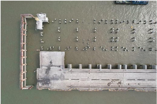
图 2 原码头面板拆除后出露的原桩位 Fig. 2 Original pile position exposed after demolition of the original wharf panel
