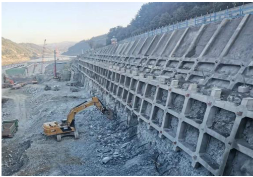
图5 “框格梁+预应力锚索”支护效果 Fig.5 Supporting effect of “frame beam+prestressed anchor cable”
